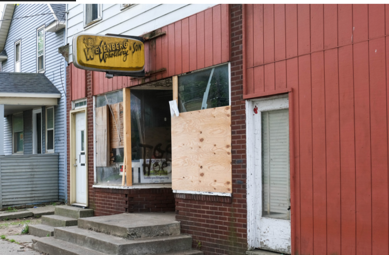
A storefront in Edison, before and after an FFE-supported facade grant.
